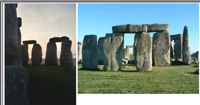
42. Early Post and Beam Construction
